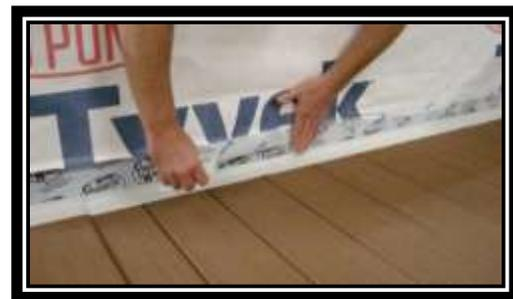
Install or reinstall siding if it has been removed for the deck installation. Install waterproofing butyl tape to the deck board (7/8") and deck post at all locations where a "through the deck support post" penetrates the deck to assure that water does not find its way through the deck to the area below.
