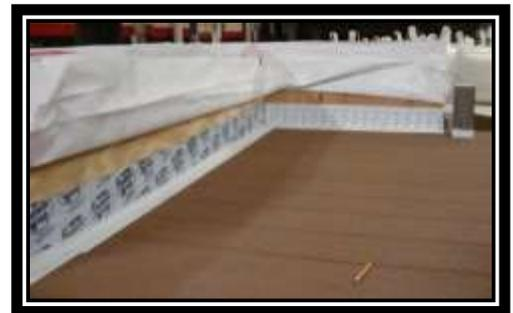
Turn the house wrap material down over the flashing and seal the house wrap material to the flashing with a sealing tape.
