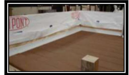
Seal the flashing to the wall under the house wrap using a sealing tape to assure that any moisture that penetrates the house wrap will not find its way behind the flashing.
