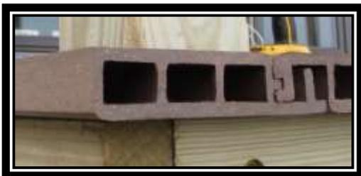
Position the first board to the deck with the fastening wing to the right side with the board overhanging the installed fascia board 9/16”.
